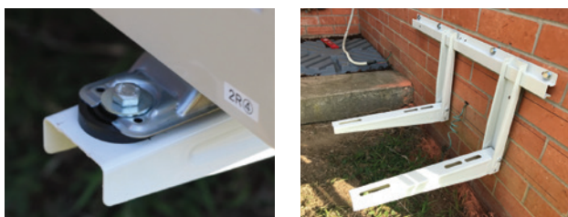
Figure 5: Wall mounting brackets.
